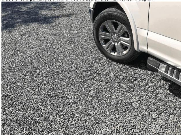
At the bottom, a filter fabric is laid to prevent the gravel from migrating, and the empty pit is filled in with gravel which is then compacted and leveled by a vehicle or heavy roller. Once the empty pavers are snapped together over the surface of the filled gravel pit, more gravel is poured over the top and pressed into the empty cells with a vehicle or heavy roller.
