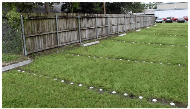
The fact that potholes cannot develop in a TRUEGRID permeable paver lot is just a by-product of their innovative design. The extraordinarily durable plastic grids keep aggregate locked into place, providing a permanent level, solid surface for vehicles to turn, brake, and accelerate on without causing damage. Water has no negative effect on these pavers either, meaning they can last up to 50 years with only minimal maintenance.
