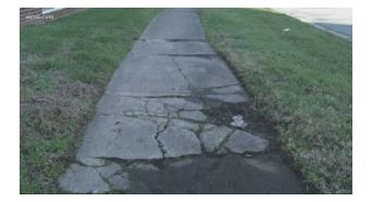
Spalling, cracking multiple areas
