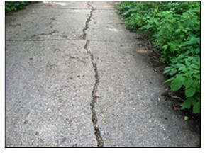
Gap in sidewalk, tripping hazard, ponding issue
